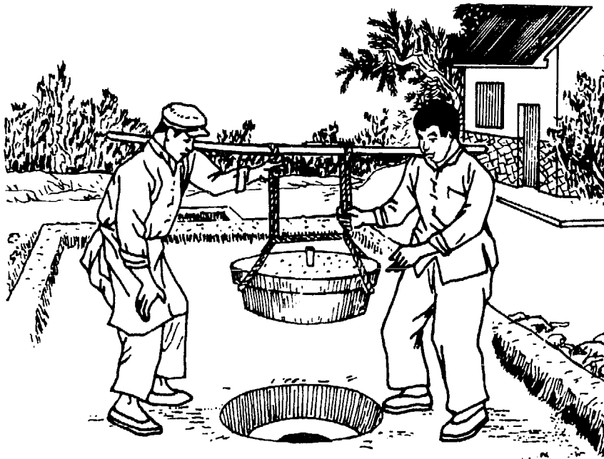
Fig. 4-23. Fitting a removable cover.
