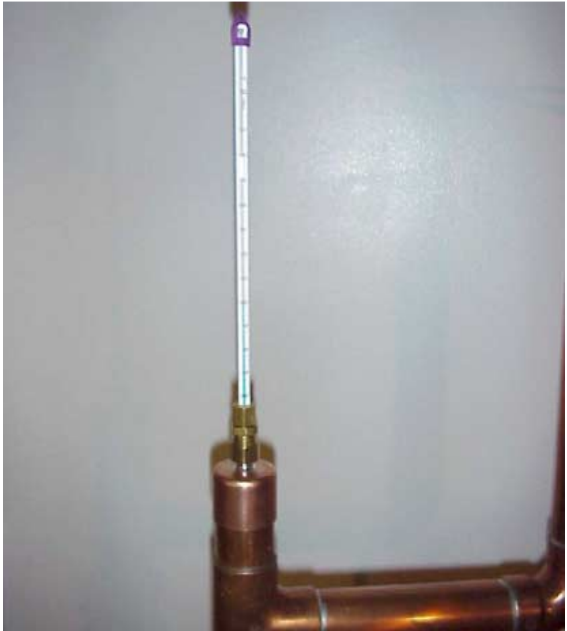
Thermometer Mounted with Compression Coupling
